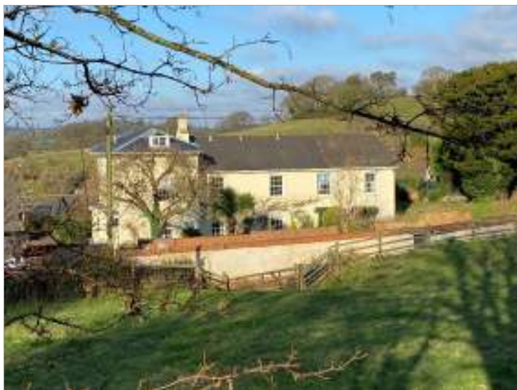
Taken from playground with site in foreground and The Old Vicarage in centre.
