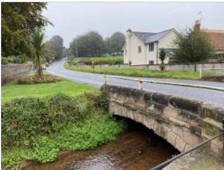
Western part of site viewed from Oakhill Bridge.
